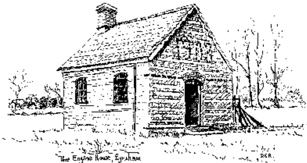
Fig.2 The pumping house in the field north of Cassington Rd. (O.S. grid reference SP 442101) was built in 1903 to supply fresh water to the tower. This building was demolished in 1982. Drawing by D.S.Richards.
