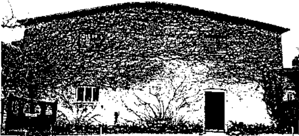
Fig.2 The low-pitched roof on the old malthouse (part of the Gables)
