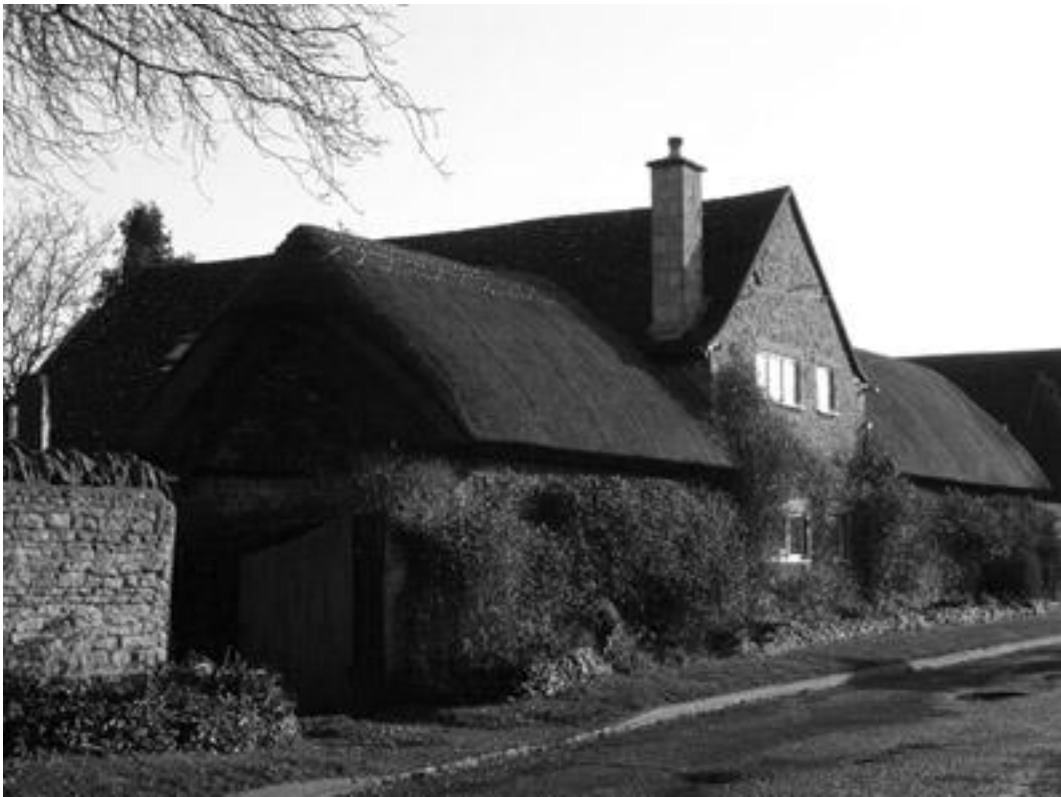
Barn after conversion
