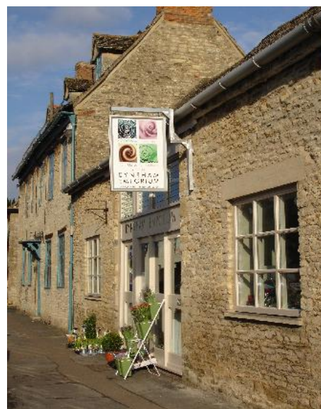
Illustration 2: Eynsham Emporium, former site of Barclays Bank
